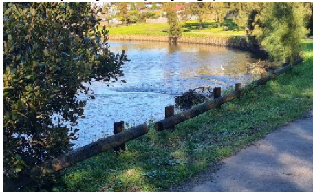
Timber post fence (half logs)
