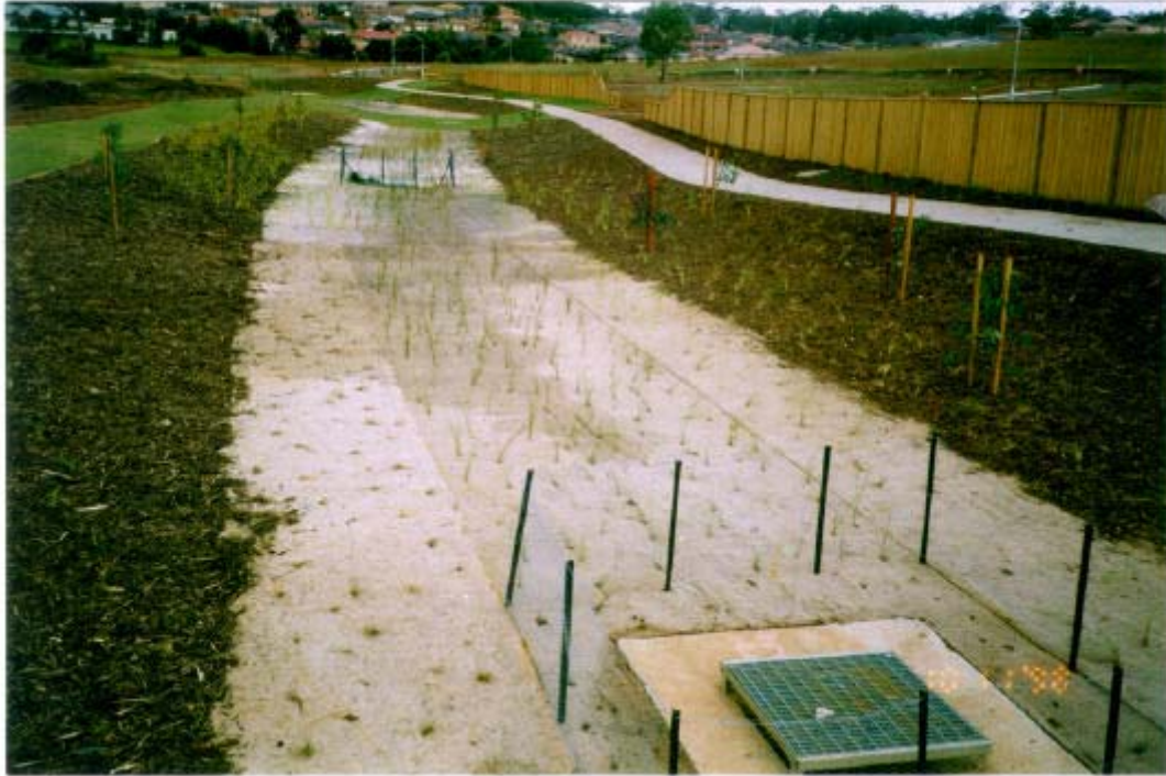
Figure 12 Recent Dechannelisation of a Concrete Lined Drain through Parkland. Works undertaken by Landcom in 1998.
