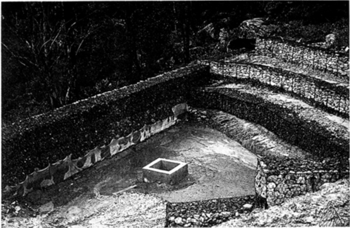
A sediment retention basin constructed on Type C soils with gabion baskets in very steep country. The structure has recently been converted to a constructed wetland.
