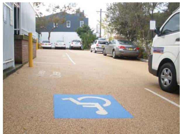
Tom Foster Community Care Centre gets retrofitted with a permeable paving car park.
