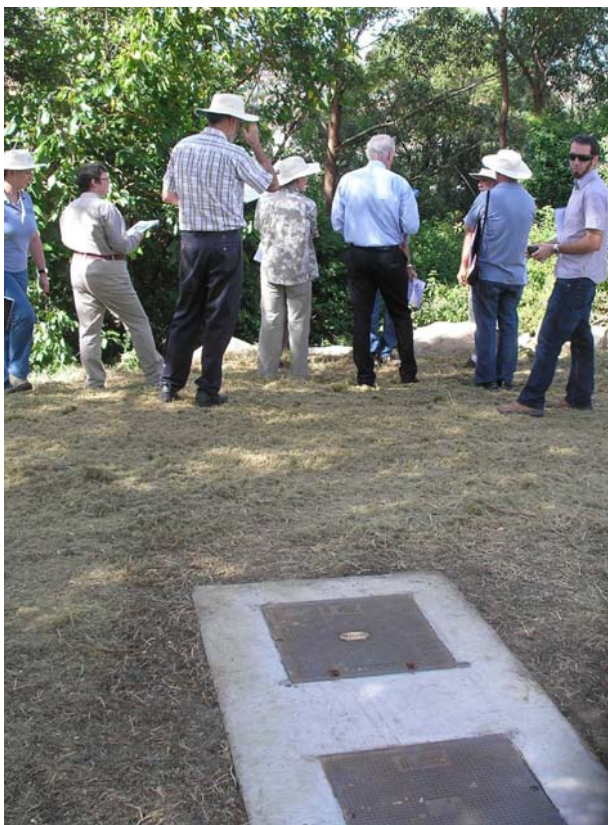
The CRUWI Reference Committee inspects a GPT installed to protect Wollie Valley bushland from impacts by stormwater coming down Highcliff Road West.
