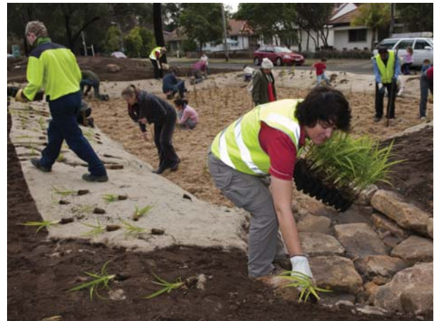
Strathfield Council designed and constructed two raingardens in the central median of Drew Street, Greenacre, with the aim of treating stormwater runoff from two residential subcatchments (1 hectare area) before it enters Coxs Creek and the Cooks River and thereby improve water quality in the Cooks River. This was the first raingarden to be constructed by council staff and, with the help of technical assistance from consultants Equatica Pty Ltd, served as a great capacity-building opportunity. Local residents also lent a hand at a community planting day held in July. The project began as one of 16 structural concept designs developed for the Strathfield South Subcatchment based on actions proposed by participants in a series of collaborative planning workshops facilitated by the OurRiver project. Funding for construction came from the NSW Government Environmental Trust grant for the OurRiver project and devolved Commonwealth funding through the SMCMA's Botany Bay Water Quality Improvement Program.
