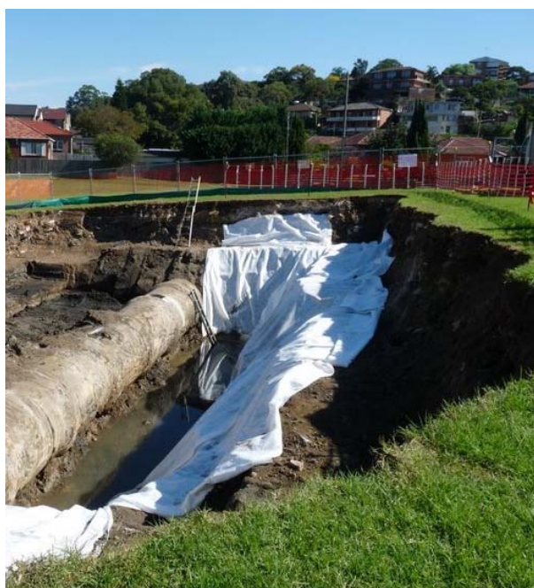
The stormwater pipe under Turrella Reserve lies exposed prior to installation of a massive CRUWI-funded gross pollutant trap to capture litter, grass clippings, leaves, gravel and sand, washed down by stormwater from the surrounding subcatchment, before they can flow into Wollie Creek. Source: SMCMA, April 2010.
