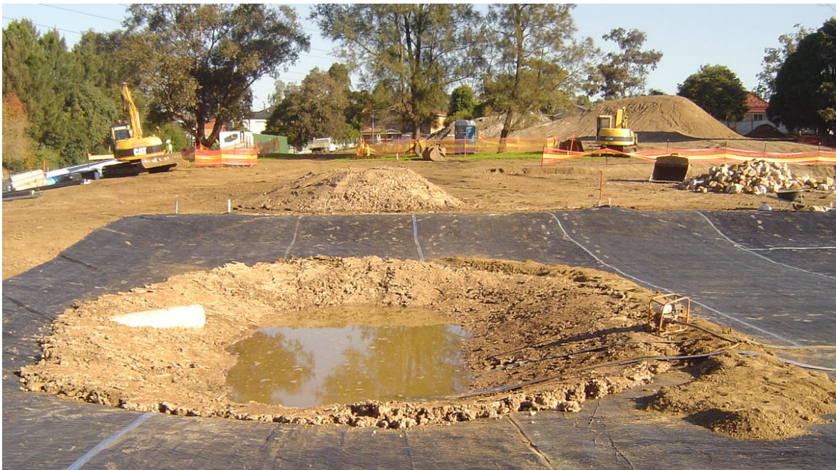
Cup and Saucer Creek stormwater treatment wetland under construction, June 2010.
