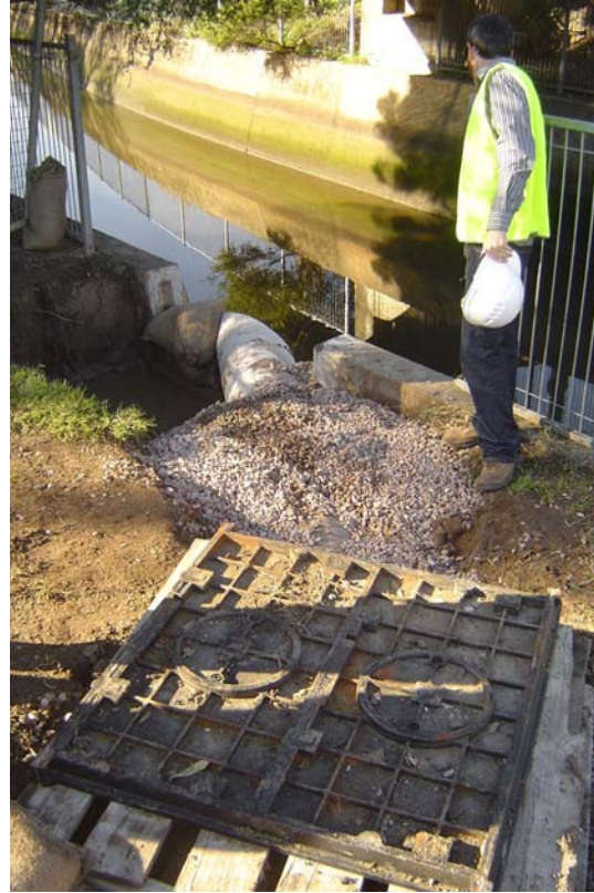
CRUWI Project Manager Phill Birtles, SMCMA, inspects the water quality monitoring pit installed at the outlet of the Cup & Saucer Creek Wetland. This and another inlet monitoring pit will be used by the CRVA Streamwatch group to sample stormwater before and after passing through the wetland, for analysis to determine the effectiveness of the wetland at filtering out nutrients and other pollutants.
