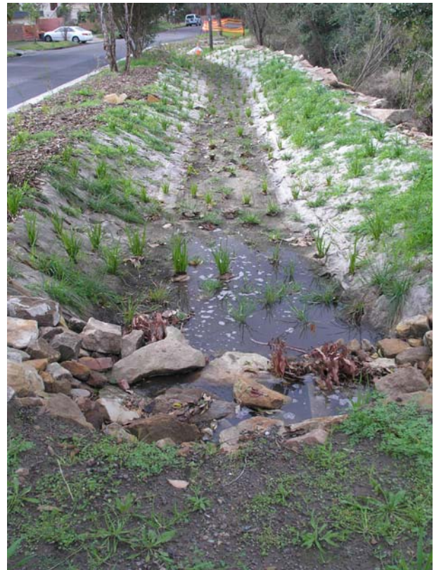
Bioretention Swale along Highcliff Road East, Earlwood
