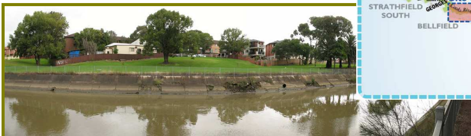
Deteriorated concrete panel on bank of Cooks River (Source: Sydney Water)
