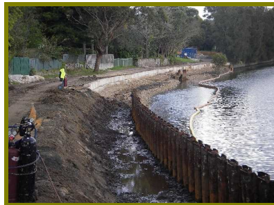
New sandstone embankments being constructed behind the deteriorated steel sheet piling, and completed works, prior to planting. Photos: DECC, 2008
