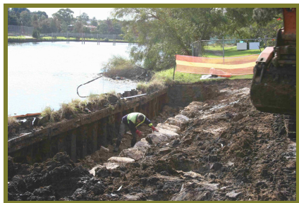
New sandstone embankments being constructed behind the deteriorated steel sheet piling, and completed works, prior to planting. Photos: DECC, 2008
