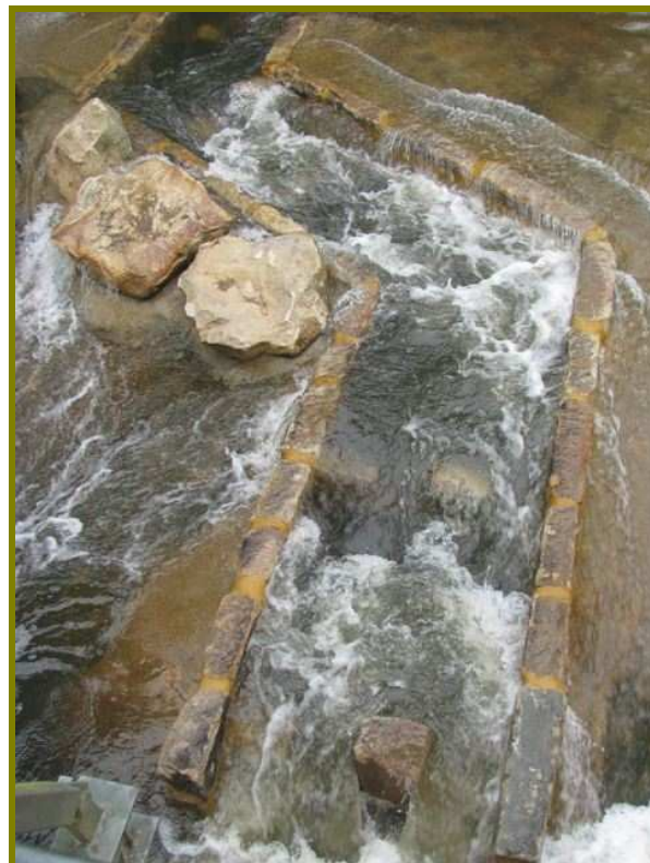
The new Wolli Creek Fishway in full flow following two days of heavy rain in February 2009. Source: Deb Little
