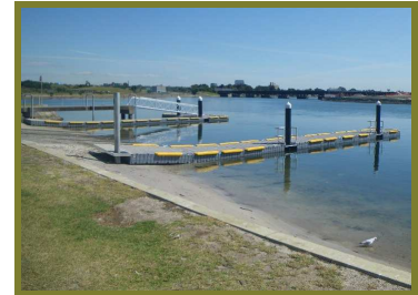
New boat ramp at Kyeemagh Boat Ramp Reserve. Source: Rockdale Council
