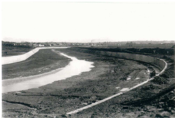
Cooks River concrete channel under construction. Canterbury, 1939 (Source: Marrickville Council)
