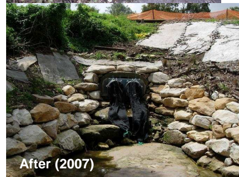
Richard Avenue stormwater outlet into Wollie Creek, before and after rehabilitation works. (Photos: City of Canterbury)
