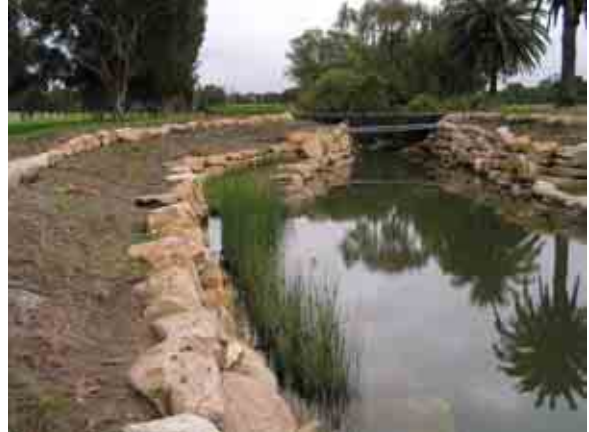
Completed bank works at Freshwater Park, April 2005. (Photo: Strathfield Council.)
