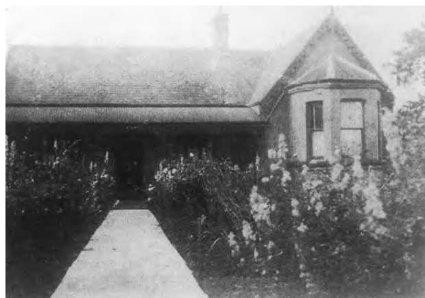
Figure 23. St Elmo, along Stoney Creek Road at Kingsgrove, date unknown.
