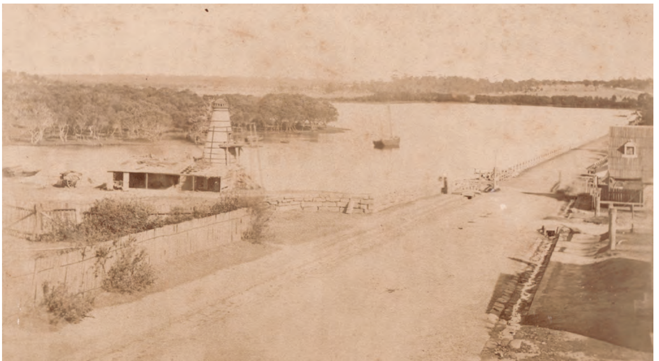
Figure 15. The conical furnace of the Tempe limekiln next to the dam around the 1870s.
