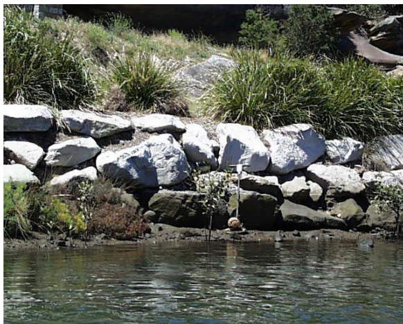
Completed riverbank restoration works near The Warren Park, Marrickville
