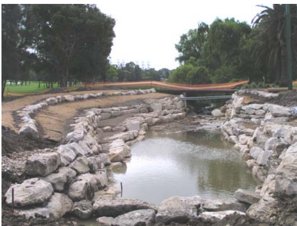
Partially completed bank restoration works, Freshwater Park, November 2004
