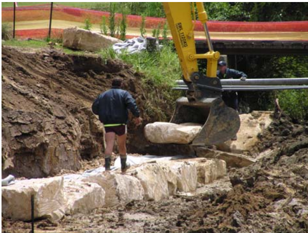
Contractors laying down toe protection, Freshwater Park, November 2004
