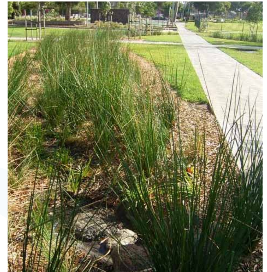
Bioretention system, Fitzroy VIC. Photo courtesy of www.wsud.org
