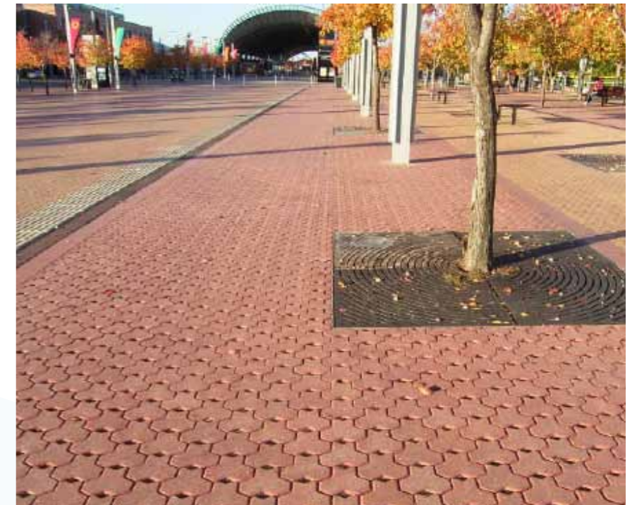
Permeable paving, Sydney Olympic Park, NSW. Photo courtesy of www.wsud.org
