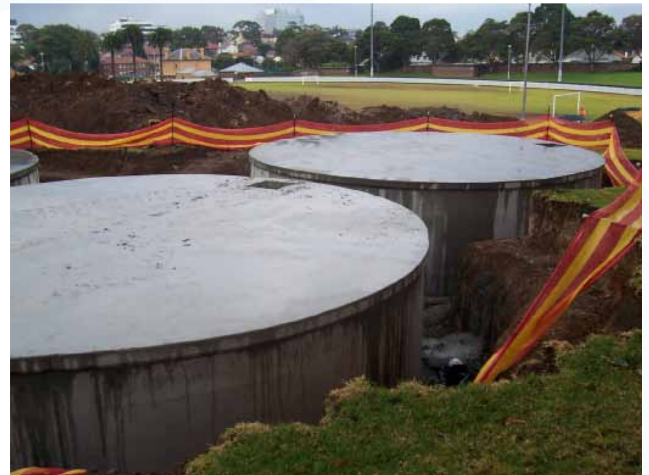
Underground water storage tanks during installation at Pratten Park, Ashfield. Photo courtesy of Ashfield Council.
