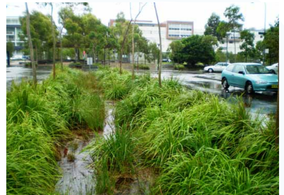
Raingarden median strip, Victoria Park, Zetland NSW. Photo courtesy OurRiver.
