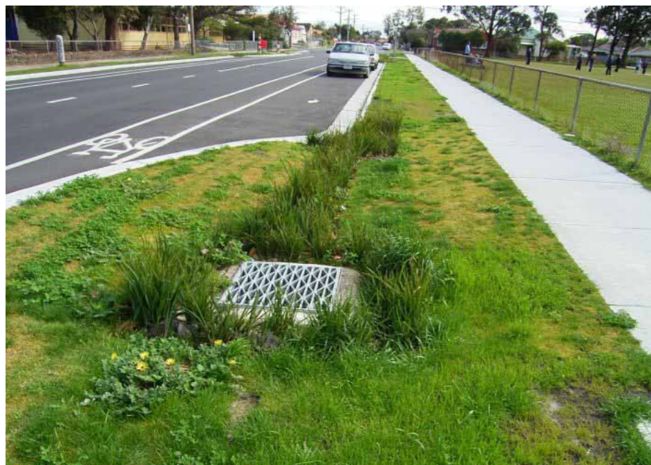
Street-side biofiltration retrofit, Kingston VIC. Photo courtesy www.wsud.org .
