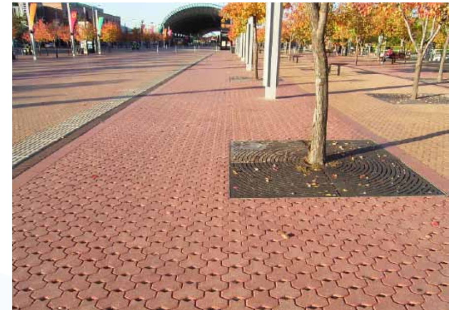
Permeable paving, Sydney Olympic Park, NSW. Photo courtesy of www.wsud.org
