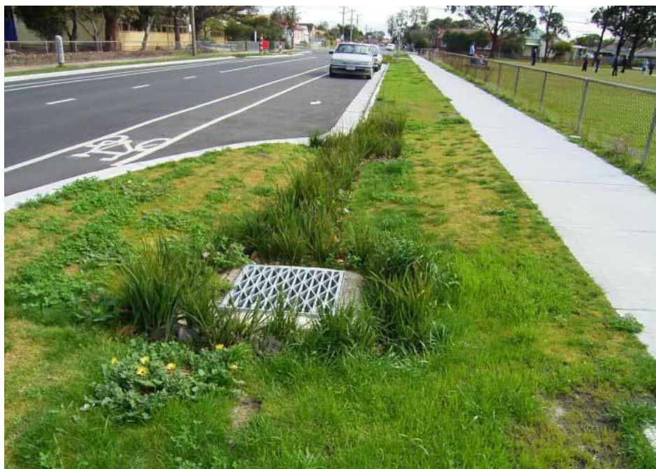
Street-side raingarden retrofit, Kingston VIC. Photo courtesy www.wsud.org
