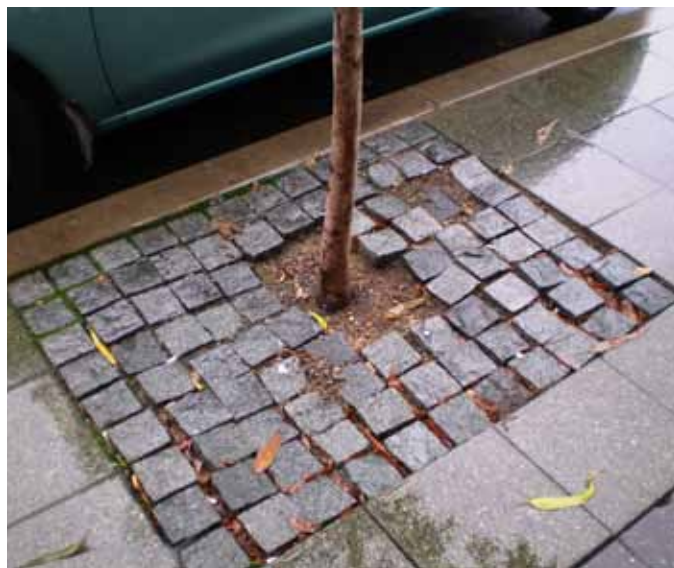
Street tree stormwater treatment (through filtration).
