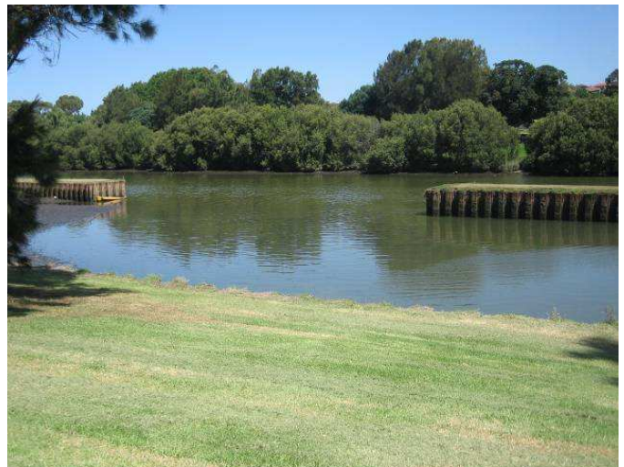
Boat Harbour on Cooks River in Hurlstone Park. Built in 1964, it became useless within 5 years as it filled with silt 2 .
