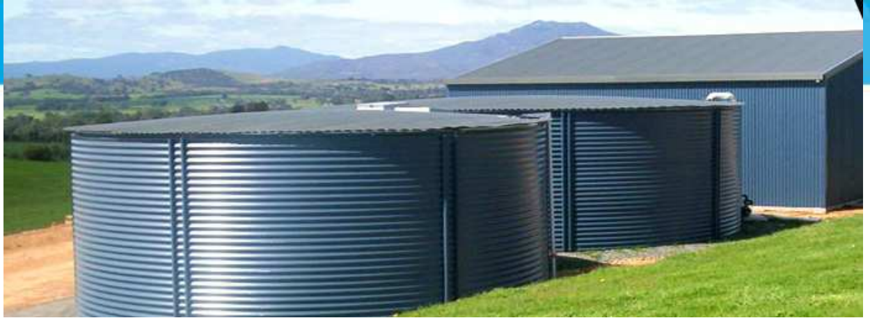
60 kl Rainwater tank – to store water for one day
