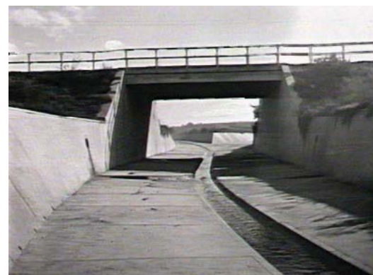
1938 - Newly completed Cooks River 'improvement' at the junction of Coks Creek and the Cooks River, Water St Bridge
