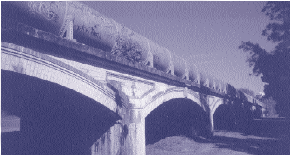
Figure 12: The South Western Ocean Outfall Sewer Crossing at Wanstead Reserve is an item of architectural heritage.
