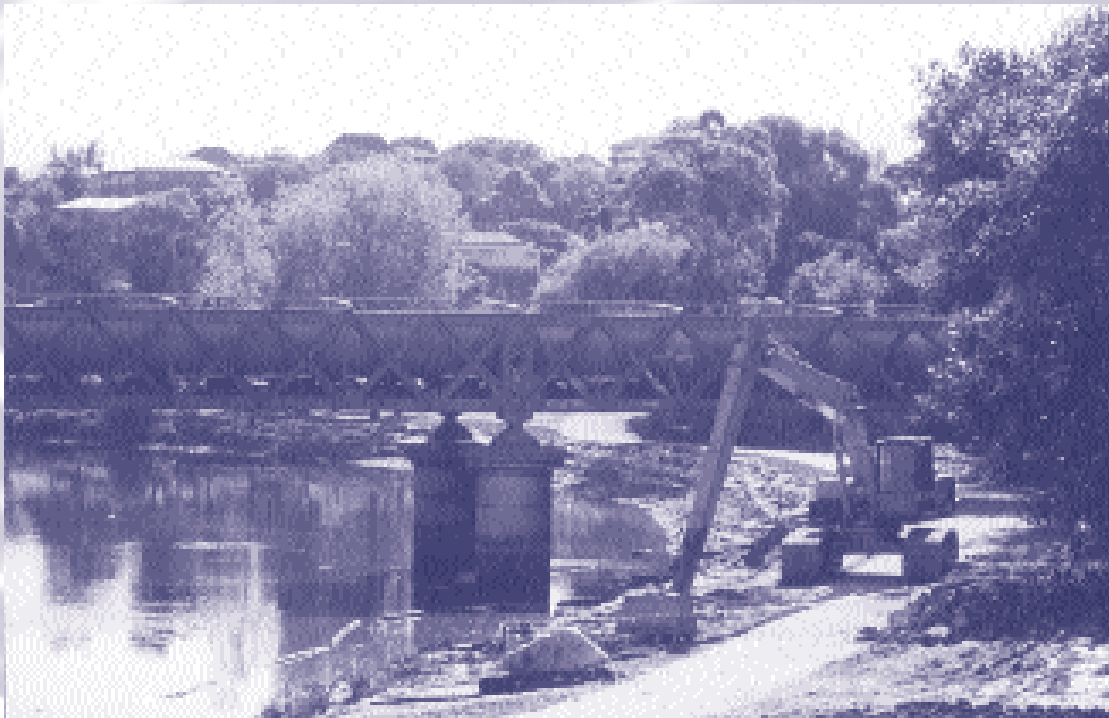
Figure 9: Restoration works in progress on the Cooks River Channel at Steel and Warren Parks, Marrickville.
